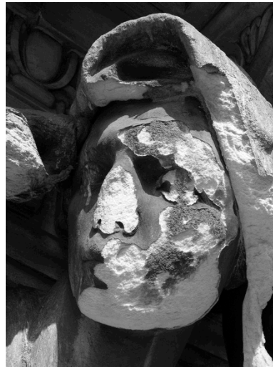
Figure 4 (above): Barnard pediment group detail showing extent of deterioration prior to treatment. Figure 5 (below): Condition were noted on assessment drawings prior to treatment implementation.
