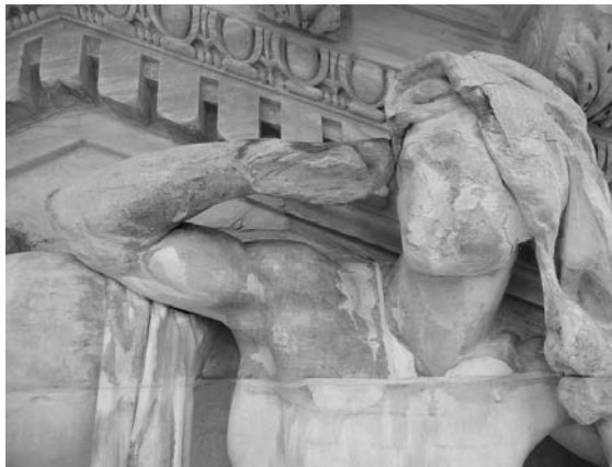
Figure 7 (below): Conditions of same figure after laser cleaning showing extent of erosion and loss.
