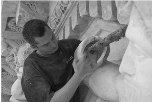
Figure 8 (above): Fitting replica casting at Barnard Pediment Group
