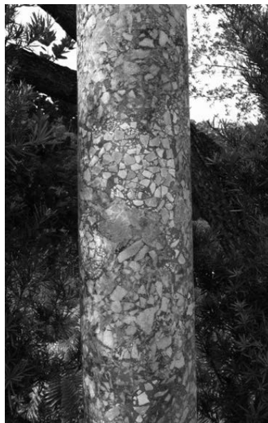
Figure 10. Example of a sample stone mosaic repair held in front of the host stone for comparison.
