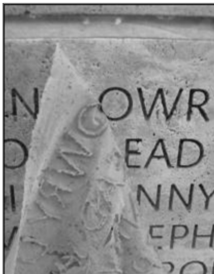
Figure 3. Prestor gel being pulled from the surface of the National Law Enforcement Officers Memorial, Washington, DC.
