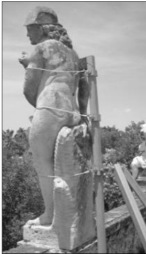
Figure 8 (left). Example of a strongback mounted to the sculpture of Pomona , an example of a sound sculpture secured to a new concrete footing.
