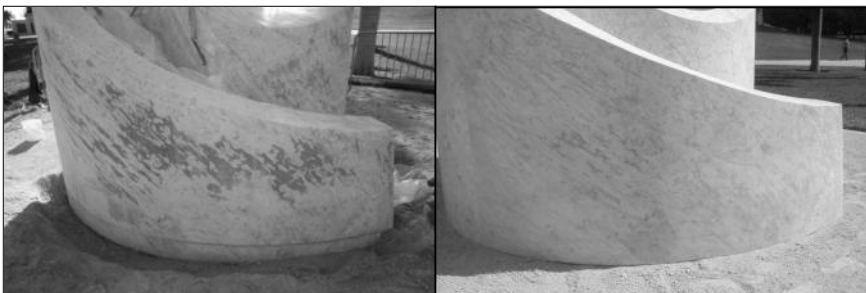
Figures 1, 2. Disfiguring biological staining before (left) and after (right) treatment with CB-4 bacteriostatic detergent.
