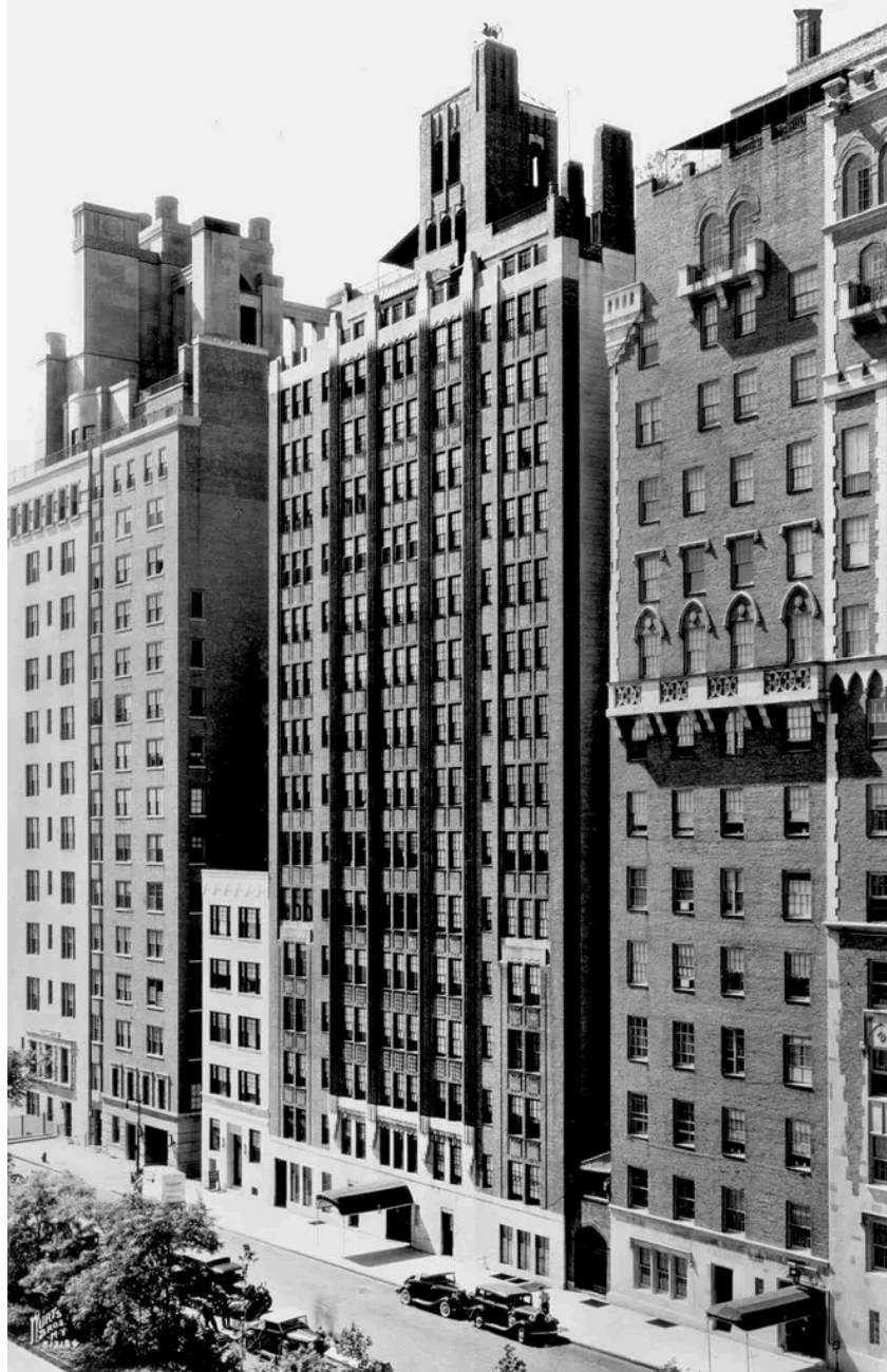
The apartment building at 7 Gracie Square, designed by George B. Post & Sons, was a project of Arthur W. Crisp, a Canadian muralist. Museum of the City of New York
