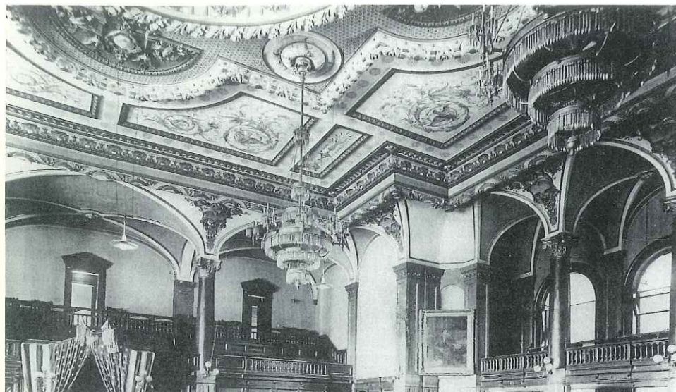
The Illinois Senate chamber in the late 19th century with its elaborate carton-pierre ornament and decorative painting, designed by architect Alfred Henry Piquenard. (Illinois State Archives)
