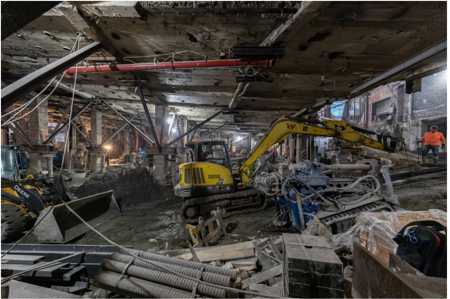
Construction underneath the theater preparing it to be lifted, in 2020.
