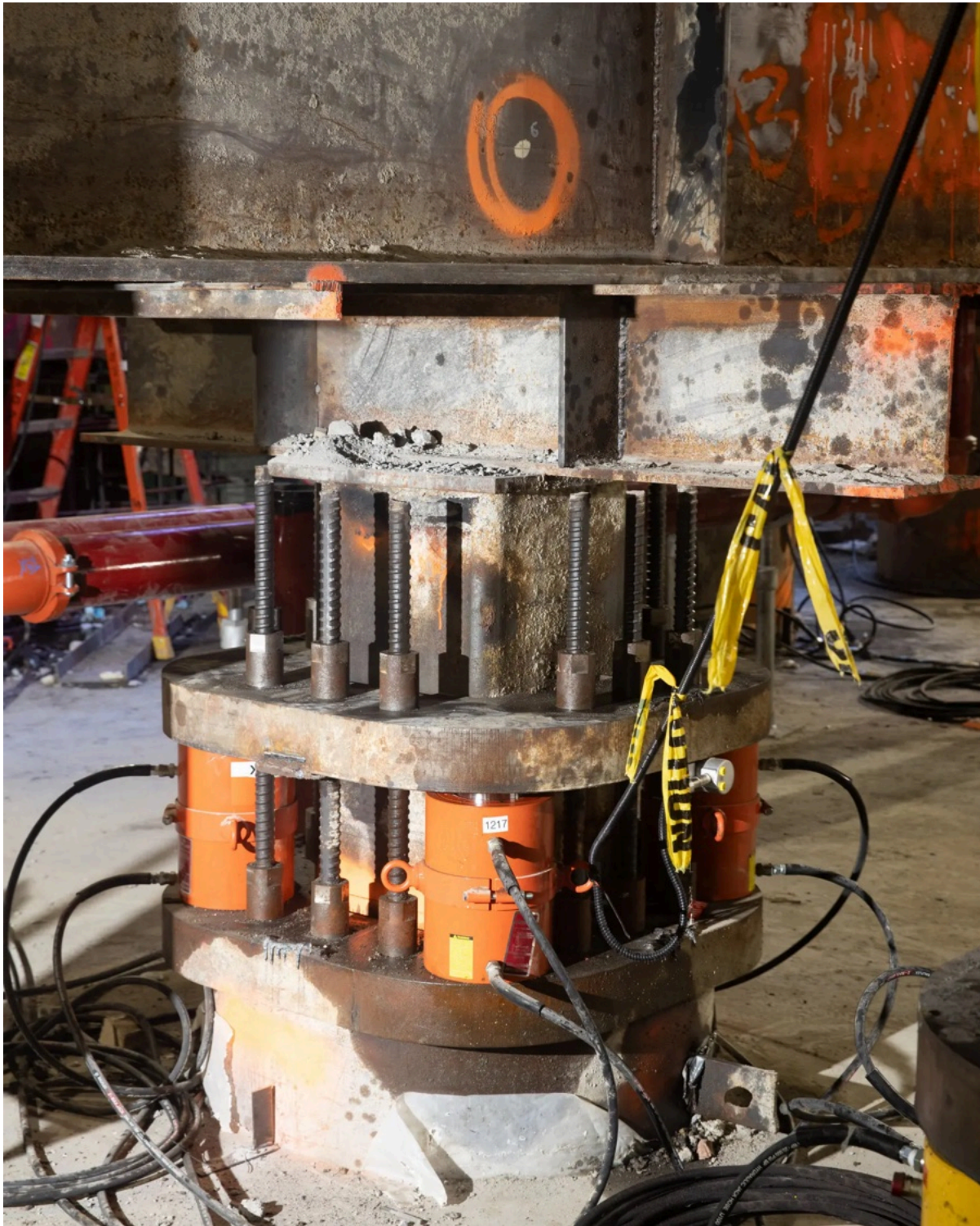
One of the lifting posts underneath the theater last year.
