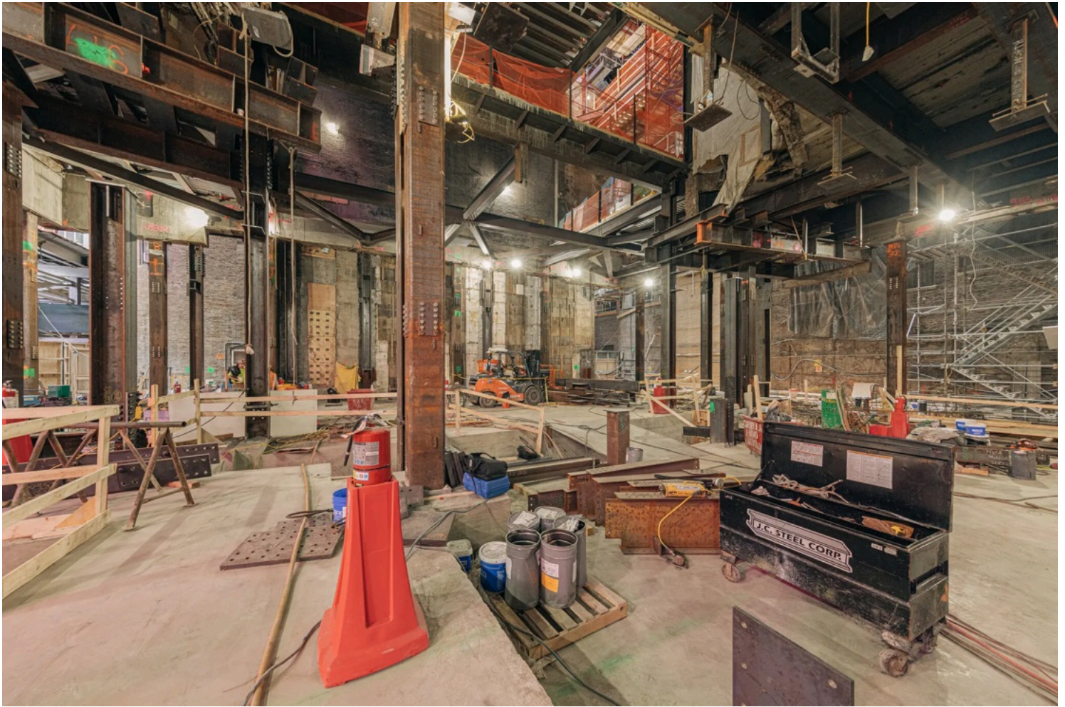
Underneath the newly raised Palace Theater, this month.
