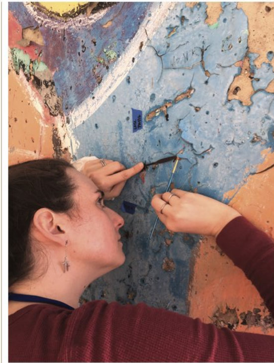
Fig. 6. Paint readhesion on the west side of the wall section, 2017.
