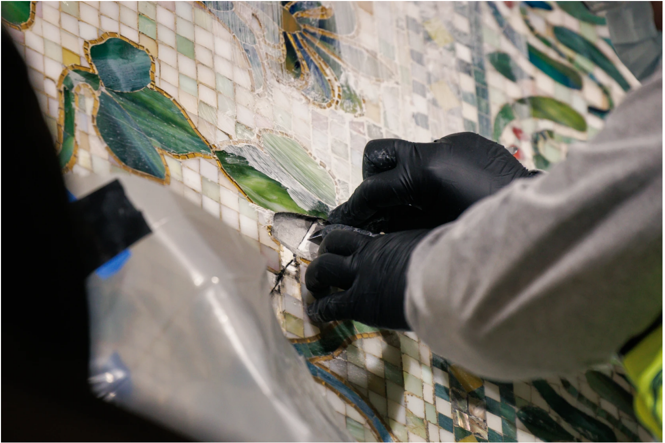
Conservator Samantha Van Kollenburg scrapes away some of the tile backing near the Preston Bradley Hall Tiffany Dome at the Chicago Cultural Center. | Anthony Vazquez/Sun-Times
