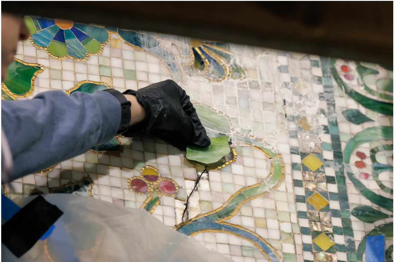
Conservator Katharine George test fits a tile near the Preston Bradley Hall Tiffany Dome at the Chicago Cultural Center. | Anthony Vazquez/Sun-Times
