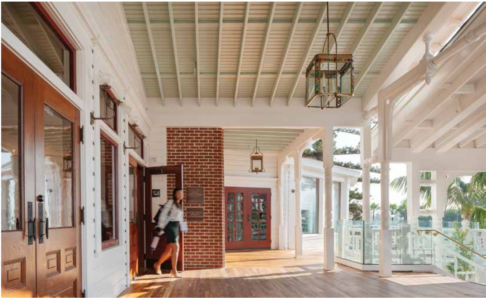
Top: Signature dark red window sashes make a crisp contrast to the restored white siding and window frames. Opposite: A new, marble-topped reception desk references original details.
